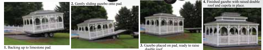
1. Backing up to limestone pad.
