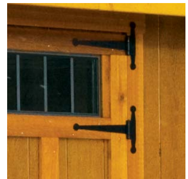
Strap hinges Decorative and functional, replaces piano hinge.
