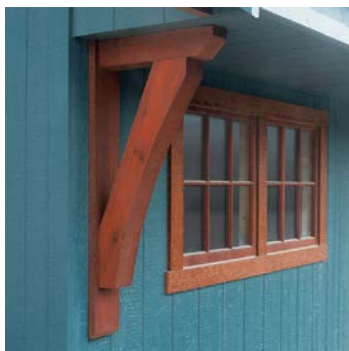
Arched Timber Brace For the extended eaves of Newport.
